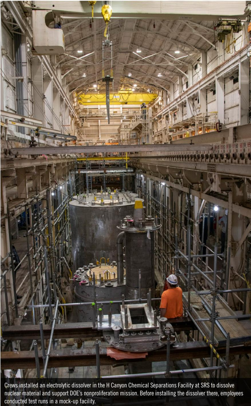
Crews installed an electrolytic dissolver in the H Canyon Chemical Separations Facility at SRS to dissolve nuclear material and support DOE's nonproliferation mission. Before installing the dissolver there, employees conducted test runs in a mock-up facility.
